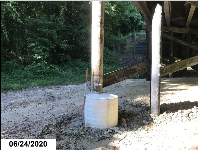
Bent 3 pile 8 replaced
