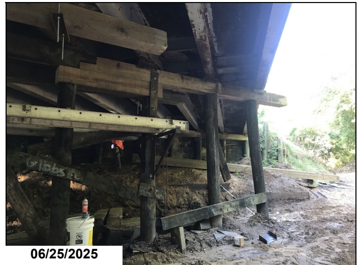
Bent 2 cap Left Splice over pile 4
