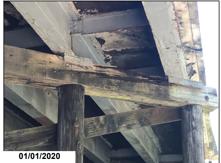
Bent 5 cap between piles 7 and 8 2019
