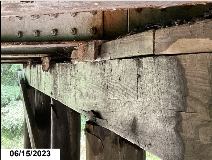
2023 - Bent 5 spacer under girder 4
