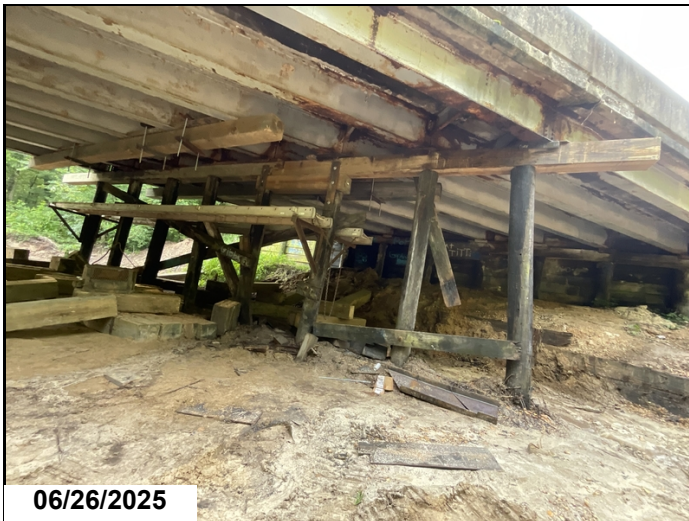
Bent 2 cap ahead side. Replaced by D10 bridge crew 6-26-2025.
