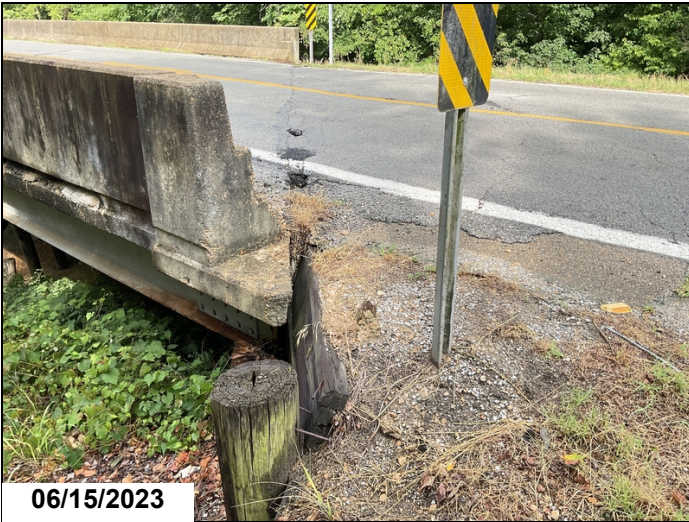
Approach at end / Bent 6 backwall
