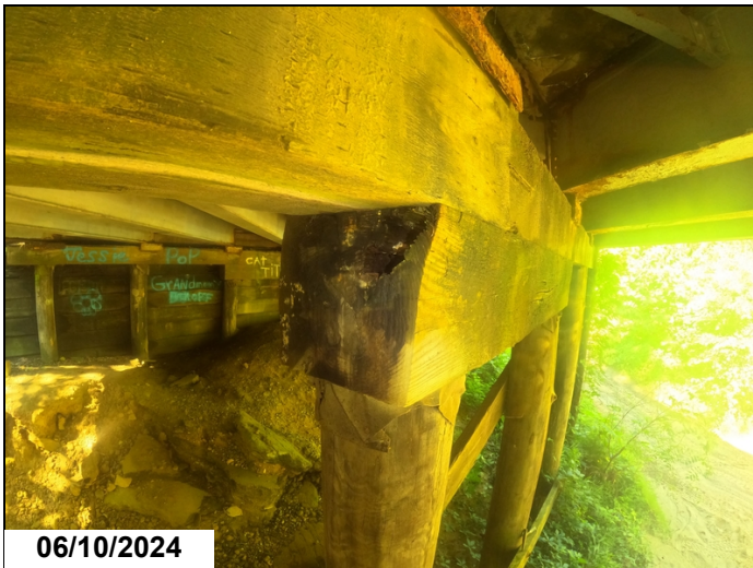
Bent 2 sub cap over pile 4
